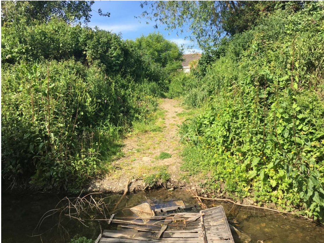
Photo 3. Looking north over the crossing area of the access road over the Three Trouts Stream.
